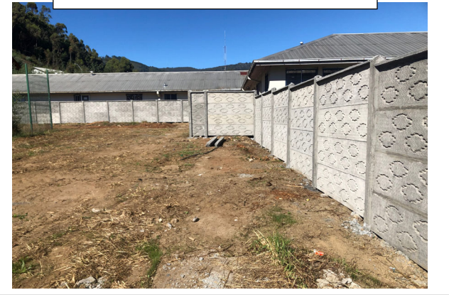
Fig.3: Cierre perimetral pandereta
