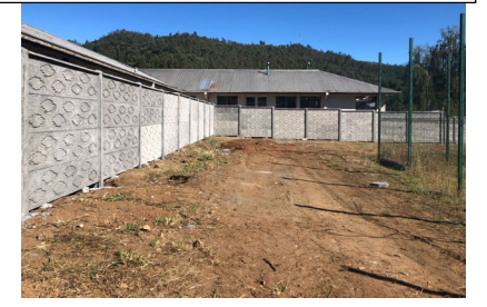
Fig.4: Cierre perimetral pandereta
