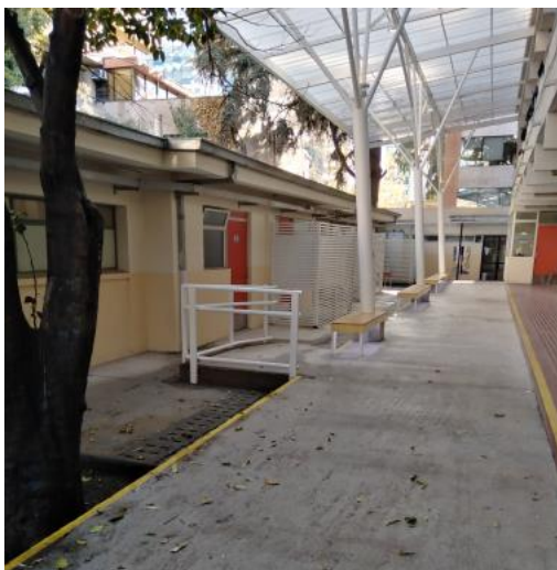
Vista general patio sector baños
