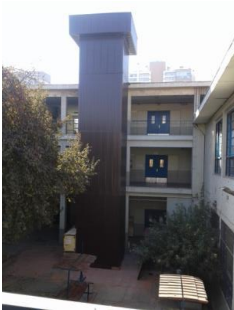
Vista general ascensor
